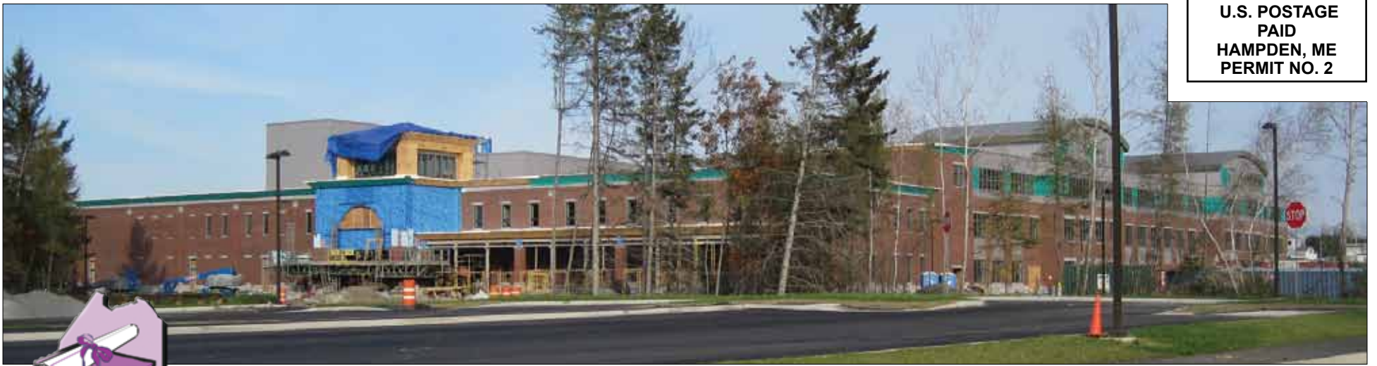
View of the main entrance to the new Hampden Academy (left center of photo) and the three-story classroom wing (right).
