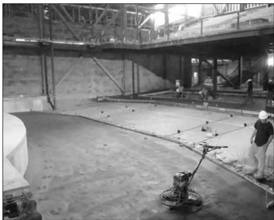
Work proceeds on the performing arts center.
