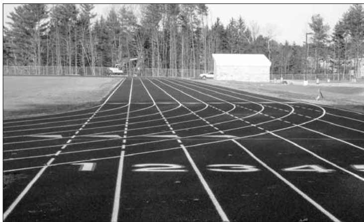
The new 8-lane track is now complete.
